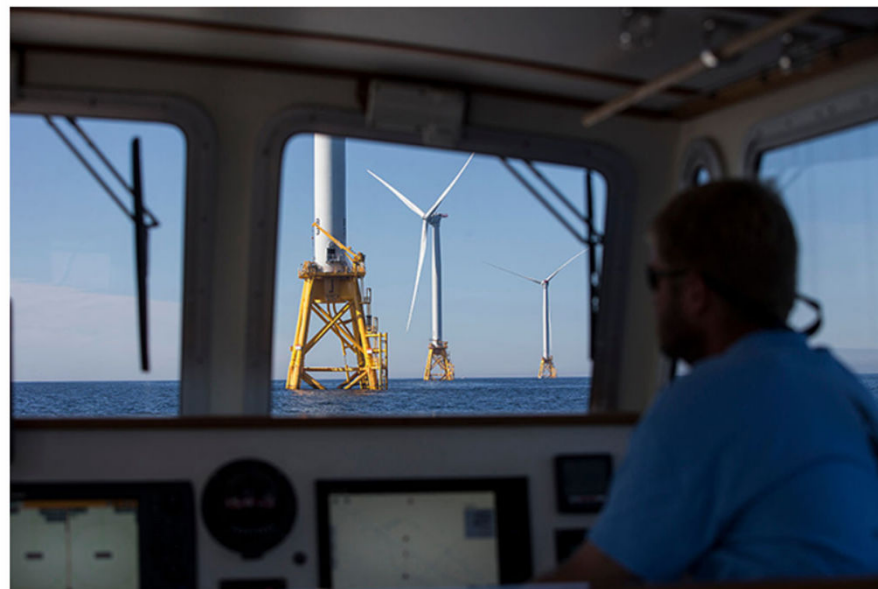
Denmark's Ørsted owns the first offshore wind project in the U.S., the 30-MW Block Island wind farm. The industry is now bracing for exponential growth.
